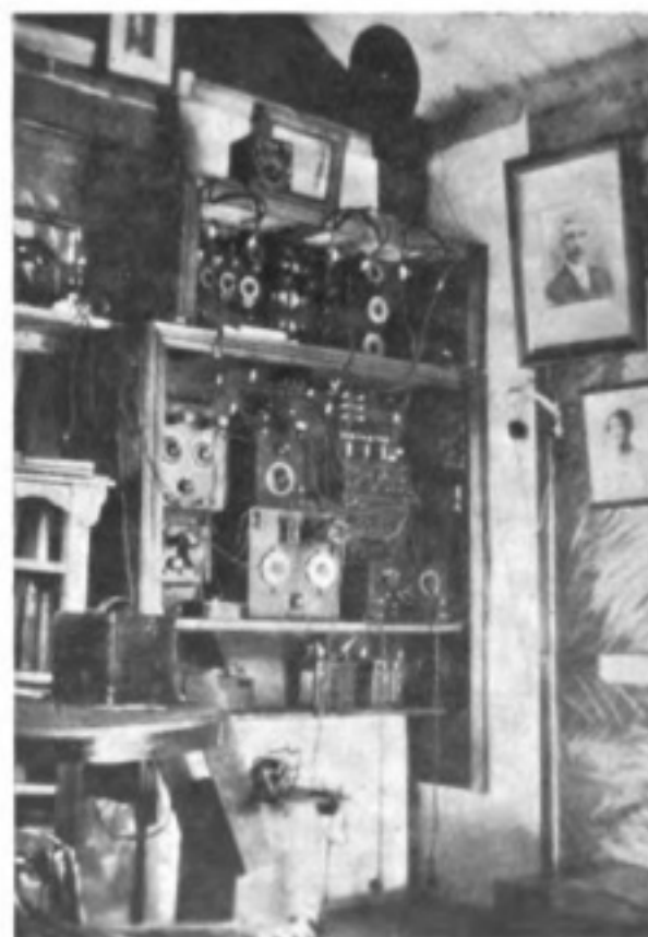
Interior view of Mr. Fudger's Station.
